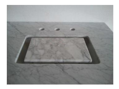
7. Leave it untouched for 12 hours for silicon/glue to set. Seal all stone surfaces with stone sealer before use. Caulk along the sinks. Consult with your local hardware store with regards to stone sealer.
